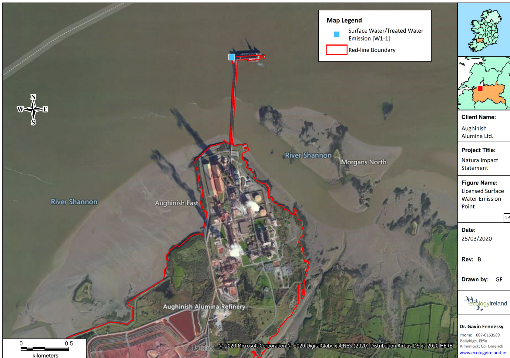
Figure 5.4.1 Licensed Surface Water emission point
